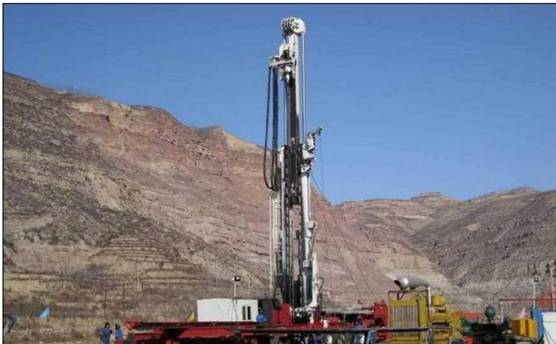
Coalbed methane drilling rig hydraulic system
