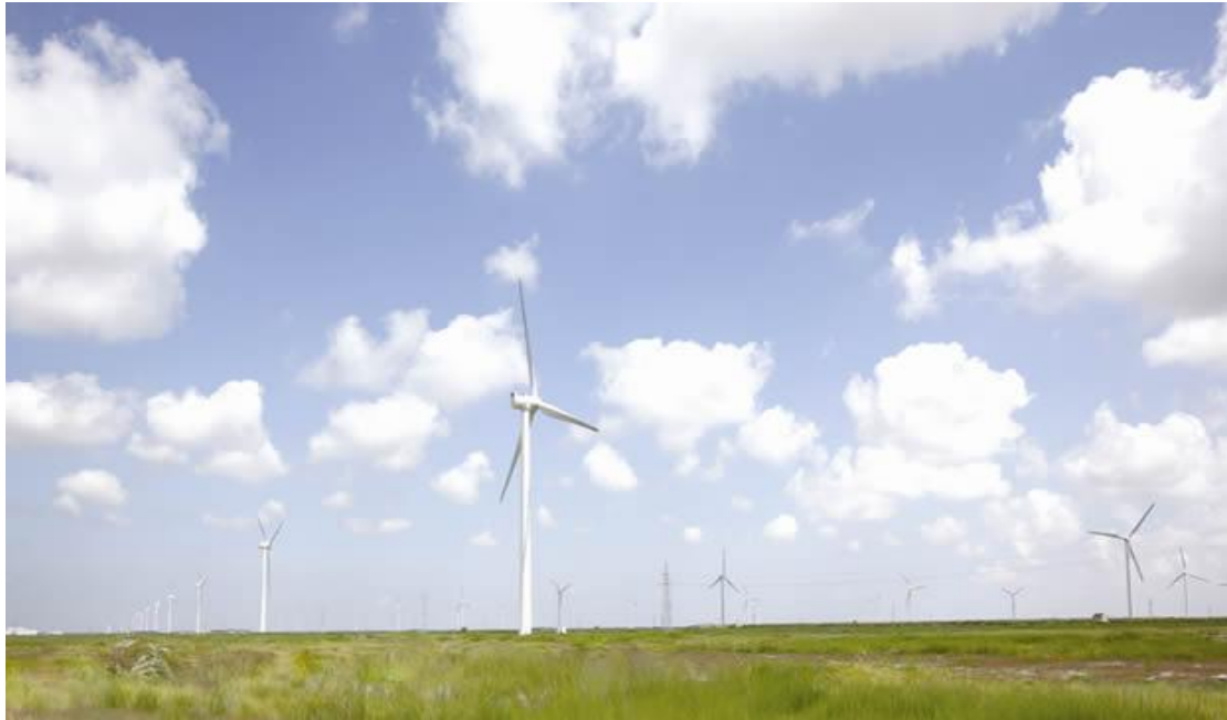
Wind Power Station in Dongtai, Jiangsu
