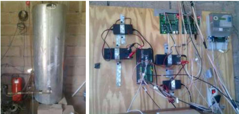
Fig. 1. Equipment inside the laboratory: (a) batteries, data loggers and wires from the sensors; (b) storage tank, circulation pump, expansion vessel, different valves and circulating ducts.
