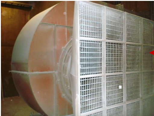
Figure 21: Fan Inlet Damper
