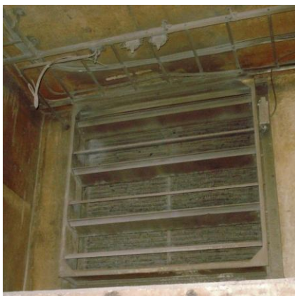
Figure 23: Wall Damper inside Fan Room
